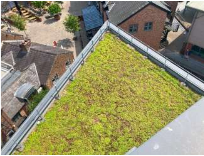
Figure 5: Extensive sedum green roof at Altrincham General Hospital
