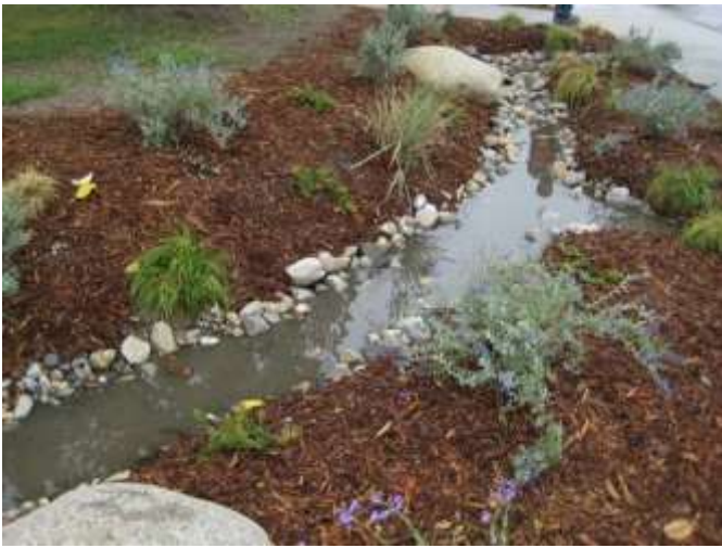
Figure 8: Bioswale acting as a channel designed to convey and concentrate storm water runoff, recharging groundwater.
